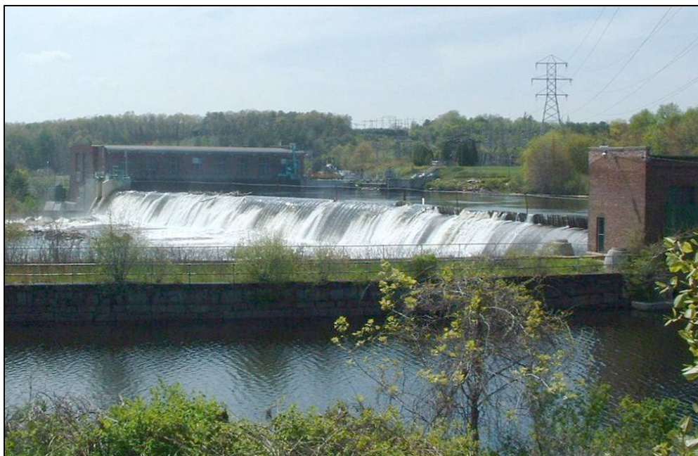
Amoskeag Dam in Manchester
