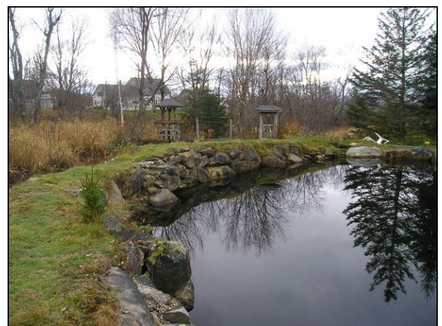
Marden Brook Hydro in Lancaster
